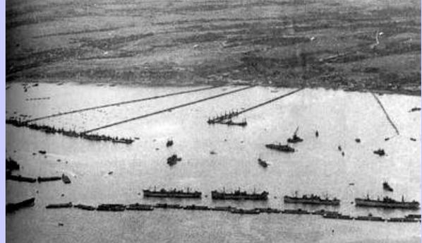
The Mulberry Harbor complex was a four-mile long breakwater, located 1½ miles from shore, and constructed of 17 scuttled de-commissioned ships and 117 concrete pontoons, each 220 feet by 60 feet by 52 feet, and weighing 3,000 to 6,000 tons.
